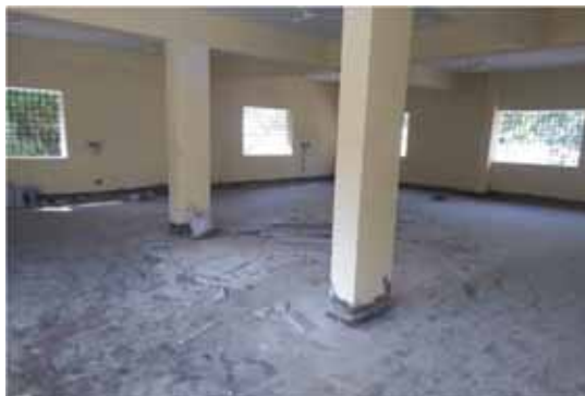
Indoor games cum gymnasium hall construction at CoA, Mandya
