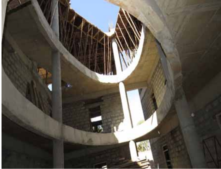
UG Girls Hostel additional block under construction
