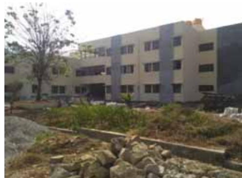
New boys hostel building being constructed containing 44 rooms at CoA, Mandya
