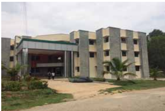
Construction of 2 nd floor of girls Hostel completed at College of Agriculture, Hassan
