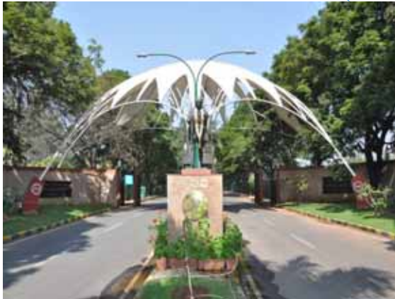
Main Entrance Gate
