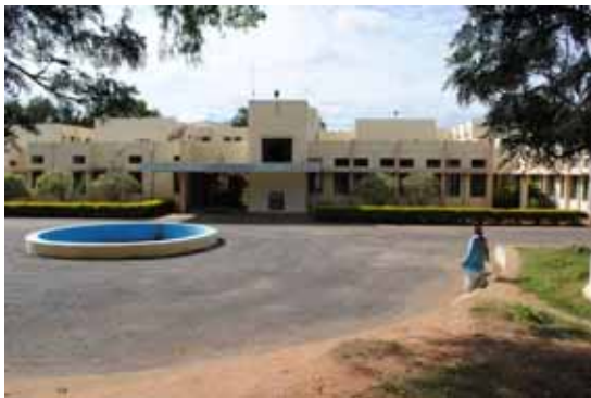
Existing college building at CoS Chintamani
