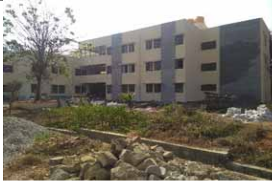
Newly constructing boys hostel building containing 44 rooms
