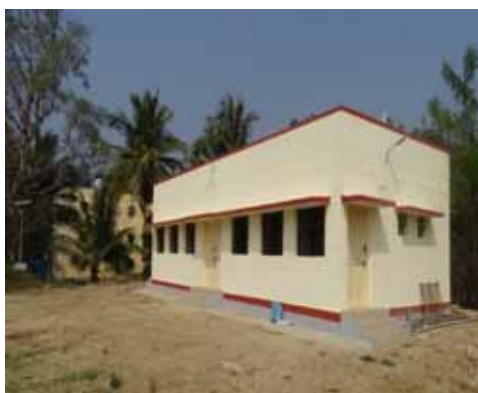
New dressing room and toilets for boys and girls constructed at the stadium, at CoA, Mandya
