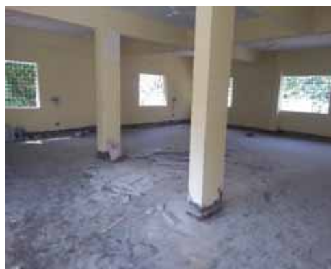
Indoor games cum gymnasium hall construction at CoA, Mandya
