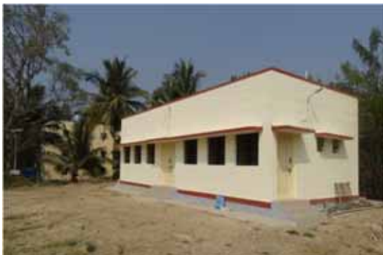
New dressing room and toilets for boys and girls constructed at the stadium, at CoA, Mandya
