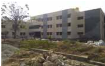
Newly constructing boys hostel building containing 44 rooms
