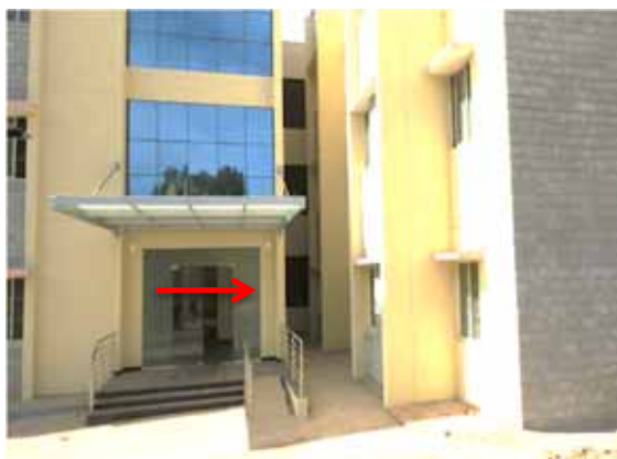
Ramps provided at the entrance of the girls hostel for the convenience of differentially abled students at CoA, GKVK
