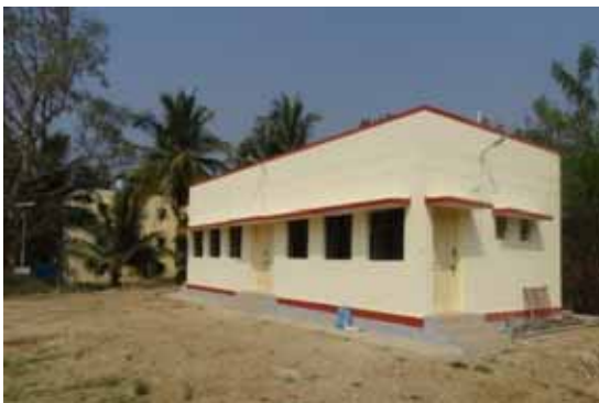
New dressing room and toilets for boy and girls constructed at the stadium, at CoA, Mandya
