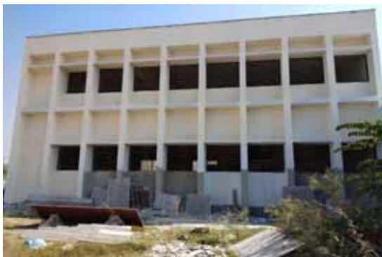
Construction of Boys Hostel under progress at College of Agriculture, Hassan
