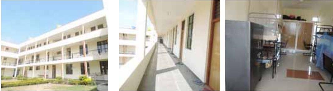
Newly constructed rooms in girls hostels at CoA, Mandya
