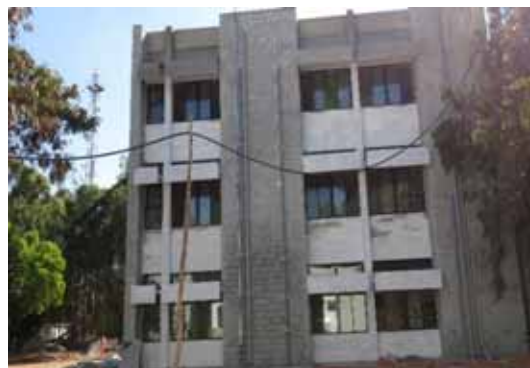
Extended East Wing, South Block (Agricultural Entomology, Genetics & Plant Breeding and Plant Pathology)
