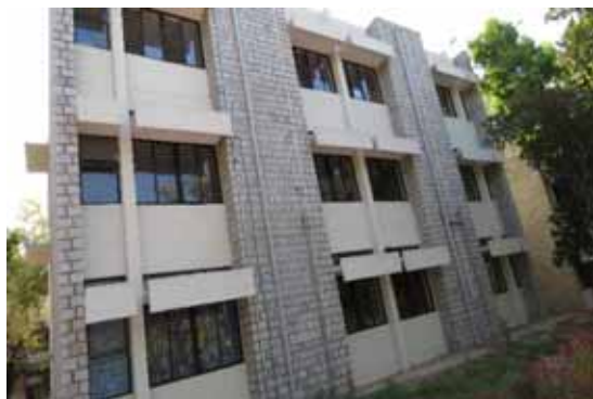
Extended East Wing, South Block (Agronomy, Seed Science & Technology and Soil Science & Agricultural Chemistry)
