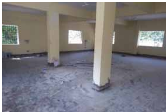
Indoor games cum gym hall construction at CoA, Mandya
