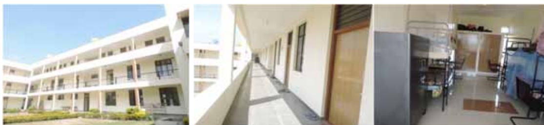
Newly constructed rooms in girls hostels at CoA, Mandya
