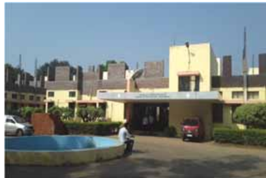
Construction of first floor to the existing college building the laboratory facility & Central Instrumentation laboratory at CoS Chintamani
